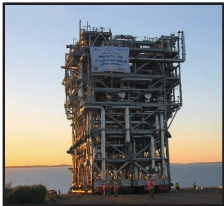
The first onshore LNG liquefaction train in the world to be constructed in modular form. The biggest module, weighing 1,800 tonnes, being transported to the North West Shelf complex at Karratha in W. Australia. Photo Courtesy: Foster Wheeler/Woodside.
