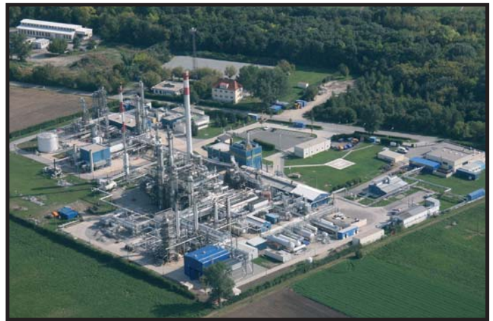
Sour Gas Plant Aderklaa I & II
