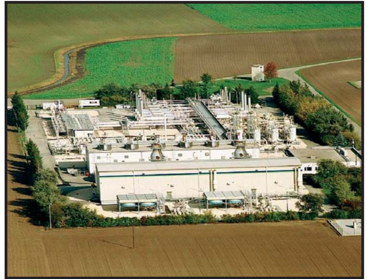
Gas Storage Facility Schönkirchen - Reyersdorf
