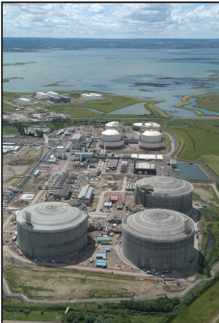
Aerial view of the terminal. Photos courtesy of National Grid
